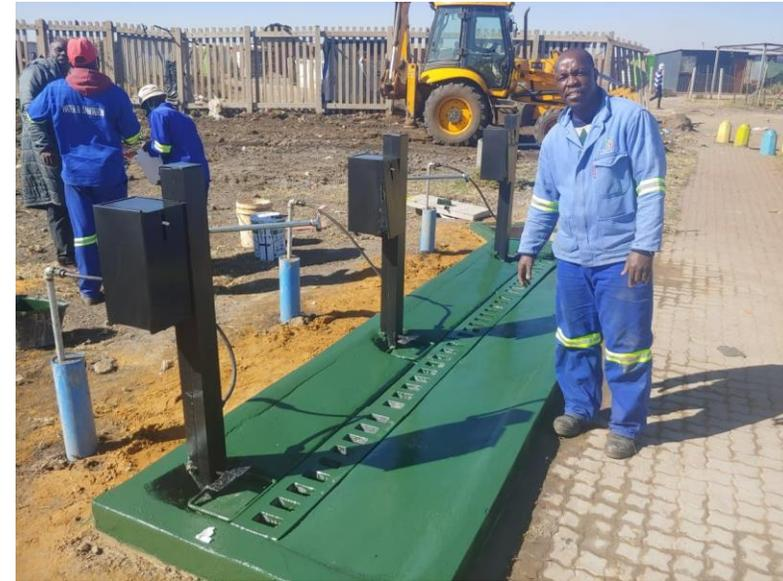
The initial 50 foot-operating public handwashing units installed in Ekurhuleni on 10<sup>th</sup> June 2020
